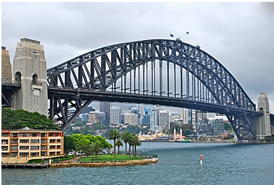
Sydney Harbour Bridge
